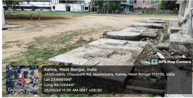
Waste water recycling through soak pit
